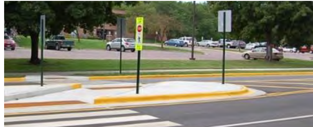
Continental Marked Crosswalk: are high-visibility pavement markings recommended for safe routes to school and other pedestrian priority areas (also note pedestrian refuges).
