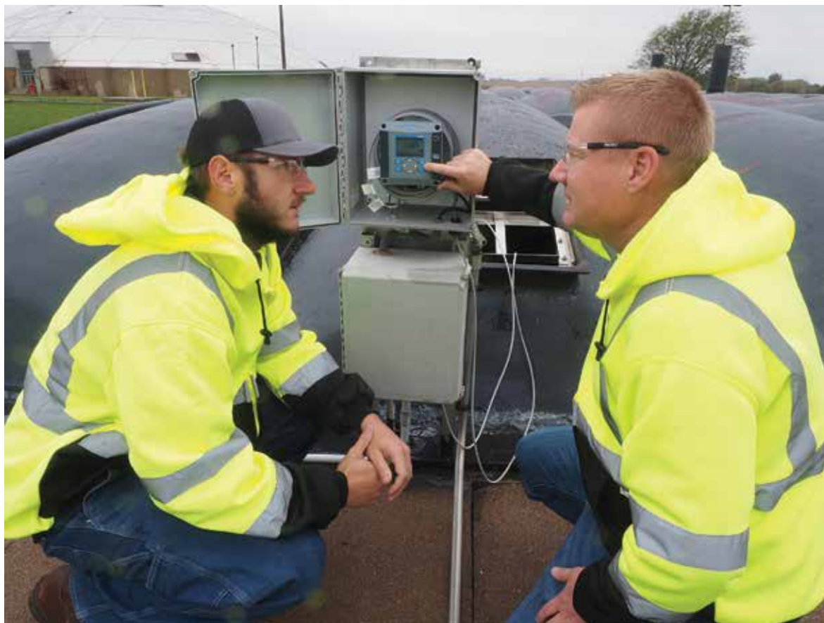
Huston, right, named Outstanding Rookie Operator of the Year by the Minnesota Wastewater Operator Association, works with Cavit Wobschall to calibrate dissolved probes using a Hach SC200 controller.
