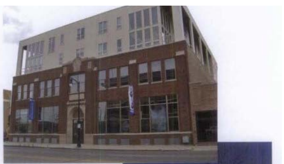
Figure 20. The height, as well as the design, of these two-story rooftop additions overwhelms the two-story and the one-story, low-rise historic buildings.
