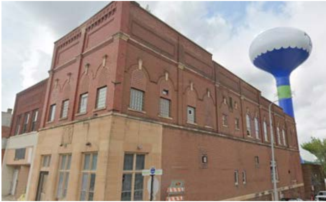
Left: View of typical flat roof shape with stepped parapet. Accessed 2024. (Google Earth) Right: Masonry and roof details. Accessed 2024. (Google Earth)
