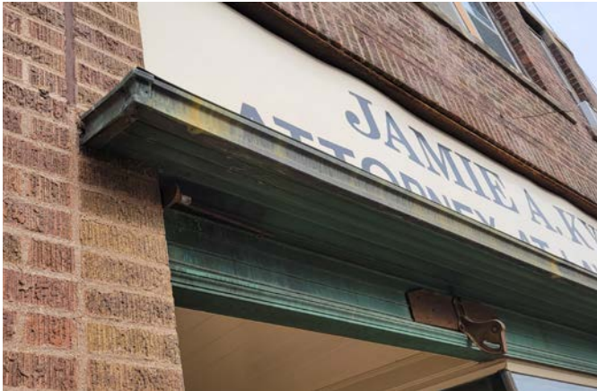
Left: Historic metal awning back band, 2023. (MacDonald & Mack Architects) Right: Historic floor tile, 2023. (MacDonald & Mack Architects)
