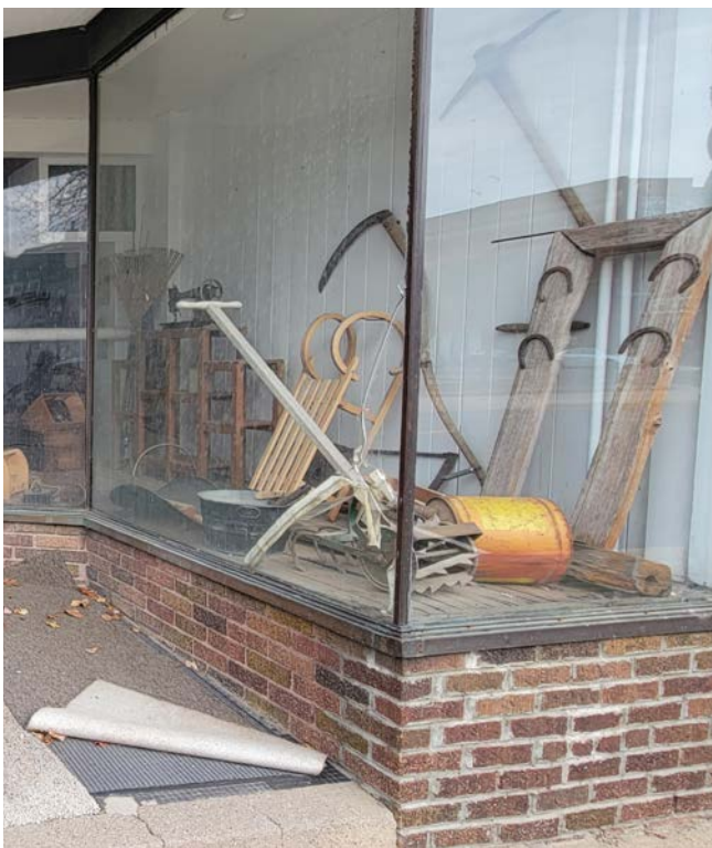
Top: Example of a close repointing match. (MacDonald & Mack Architects) Middle: Example of a poor repointing match. (National Park Service) Bottom: Historic storefront framing, 2023. (MacDonald & Mack Architects)
