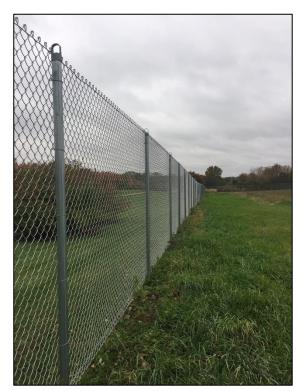
**Photo 5:** View of the airport perimeter fence along West Hammer Road. Note that the bottom of the fence is not flush with the ground, which enables small- and medium-sized mammals to enter the AOA.
